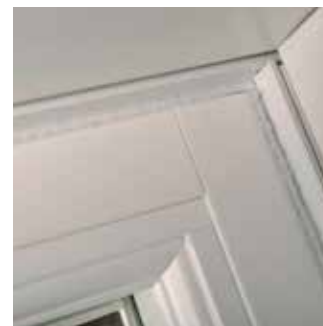
Full mechanical joints
